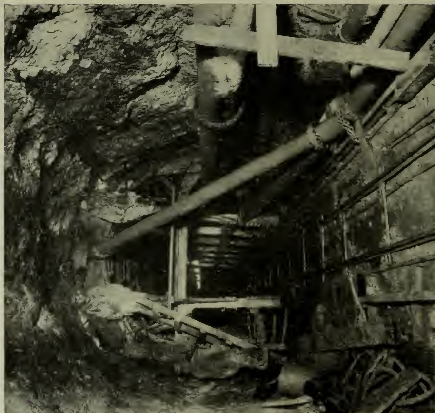
Placing Steel Forms.
